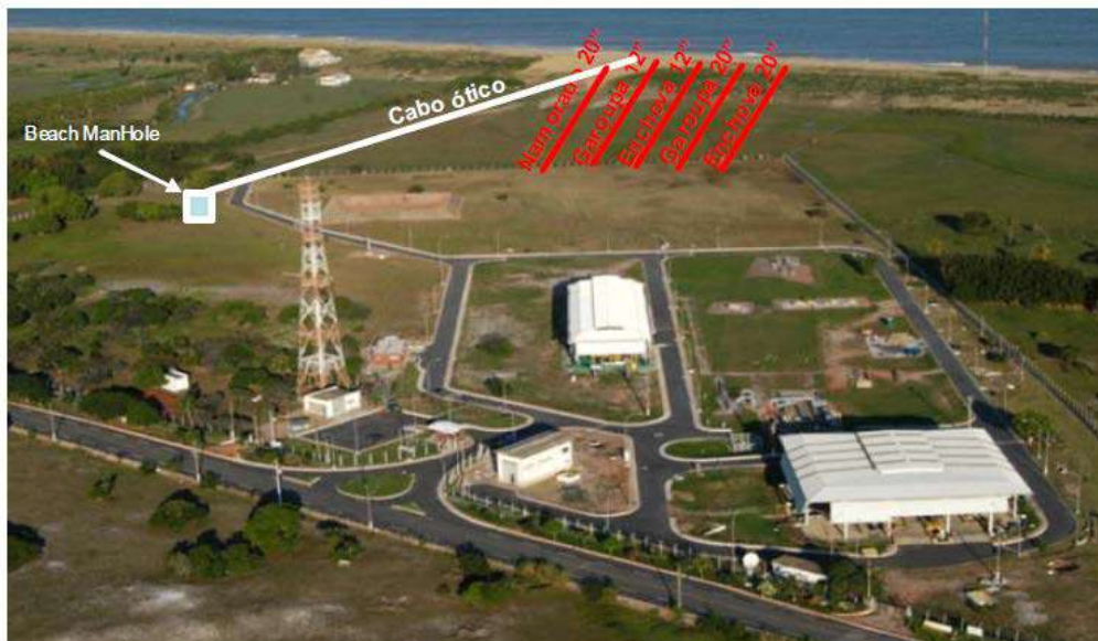
Aerial photo of the Barra do Furado Terminal (Point A) highlighting the beach section chosen for the installation of fiber optic cable
