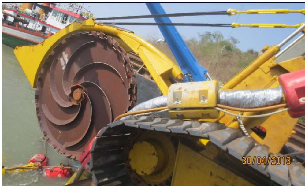
MACRO PTM for FOC laying and trenching operations
