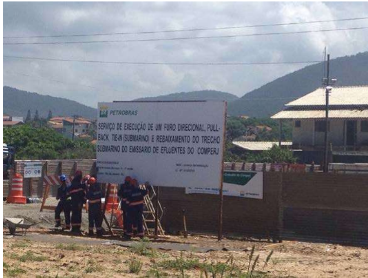
HDD onshore location
