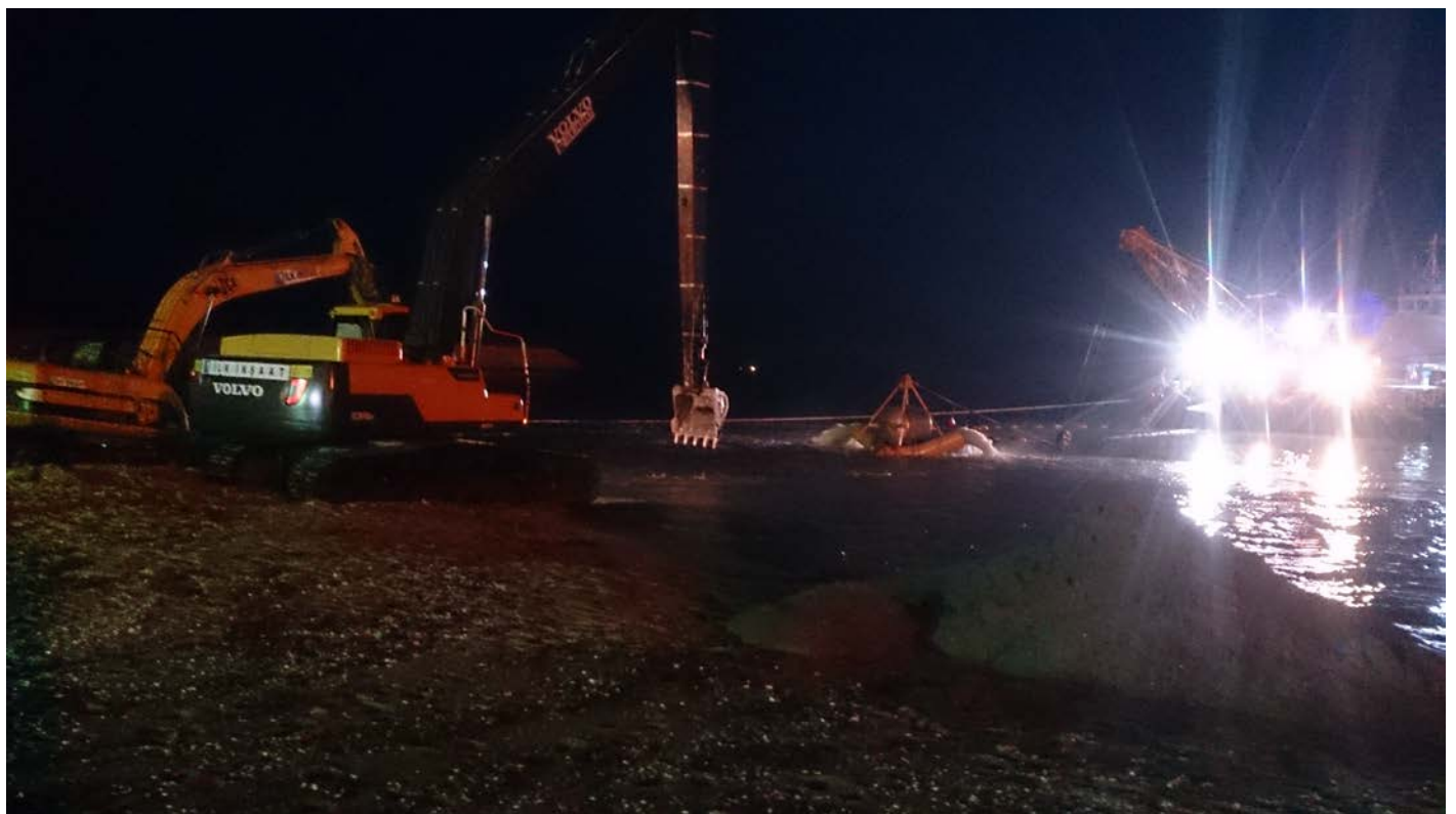
The shore approach operations
